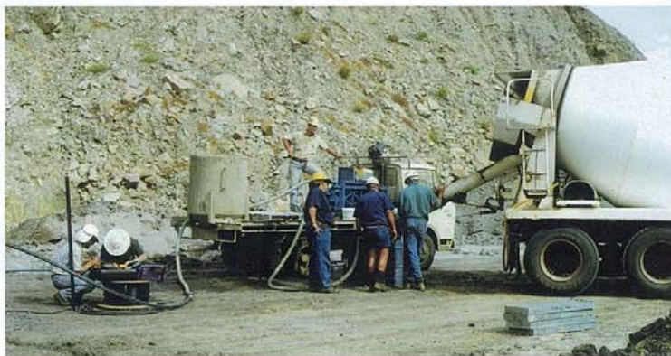
The drill string and bit were navigated sub-horizontally towards the target gas production well situated approximately 1200 m from the test drilling site. Image: CSIRO.
