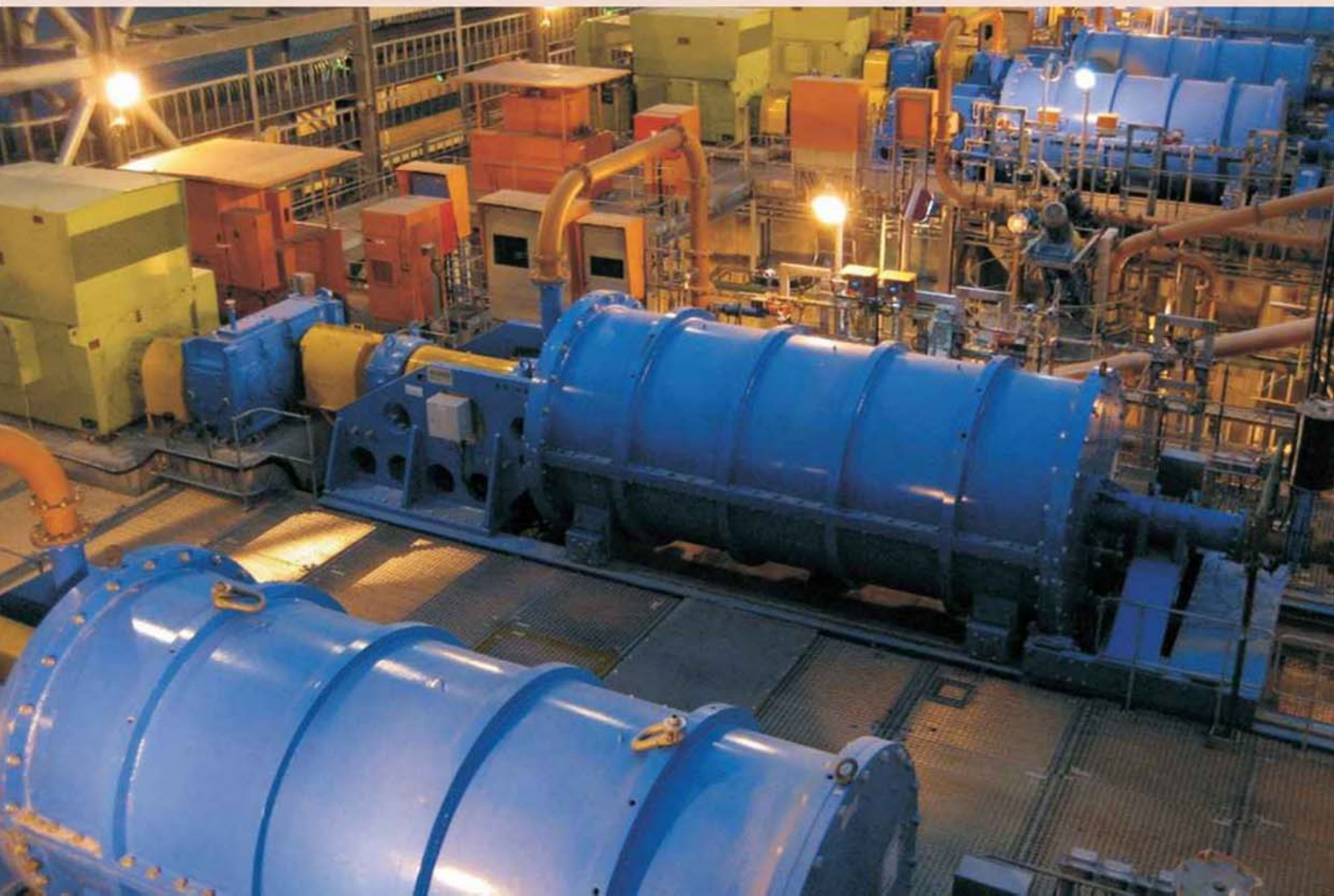
Installation for Waterval Retrofit .
