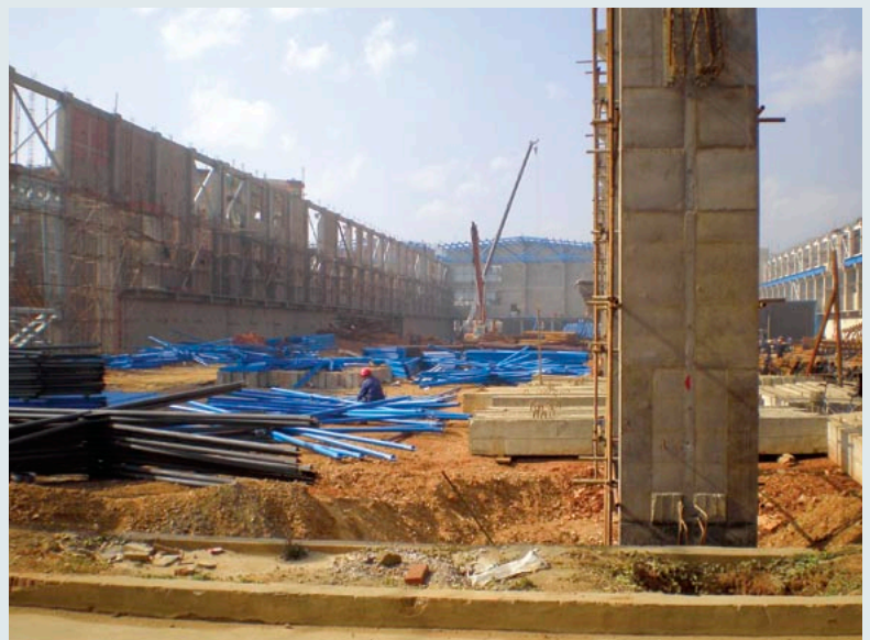
Civil Construction of Yunnan Copper's new 180ktpa copper refinery tankhouse
